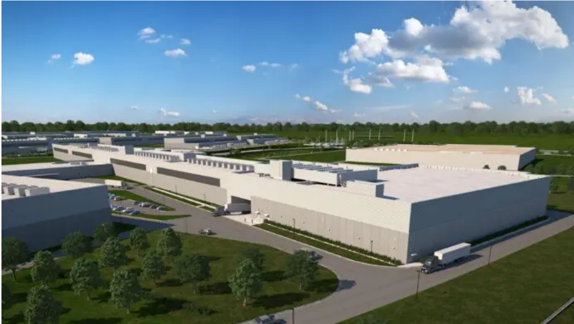
Facebook Data Center Fort Worth courtesy photo
