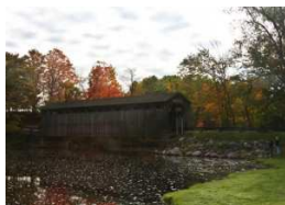
Fallsburg Covered Bridge near Lowell, Michigan
