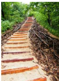
An ingenious solution to prevent dune erosion
