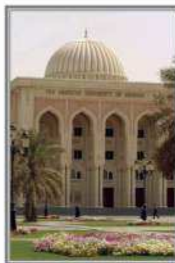
Figure 1.1 AUS Main Building
