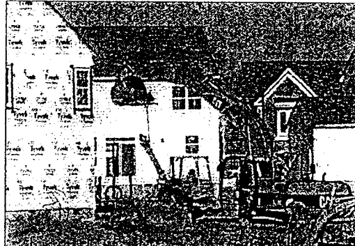
Burgeoning property values throughout Worcester County have made it difficult for average income earners to buy homes in the area. Above, construction crews continue to work at Bertie's new Decatur Farm community, a 128-unit residential project with new home prices starting around $263,000. Photo by Benjamin Hunt
