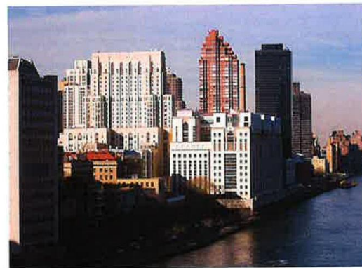
New York–Presbyterian Hospital in New York City is one of the world's busiest hospitals. Pictured is the Weill-Cornell facility (white complex at the center).
