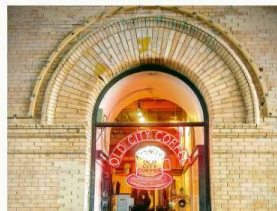
READING TERMINAL (PAD)
