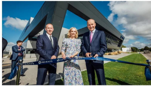
Moderna recently unveiled its new gene therapy manufacturing facility in Shannon, Ireland, on September 16, 2022, with Irish Prime Minister Michael Martin in attendance. (Source: Moderna)
