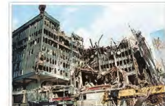
6 WTC, one of the partially collapsed World Trade Centre buildings.
