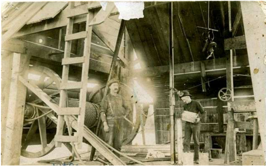
Pouring nitro into a canister to prepare a "shooting" of a well drilled using a cable-tool rig powered with a nearby steam boiler.
