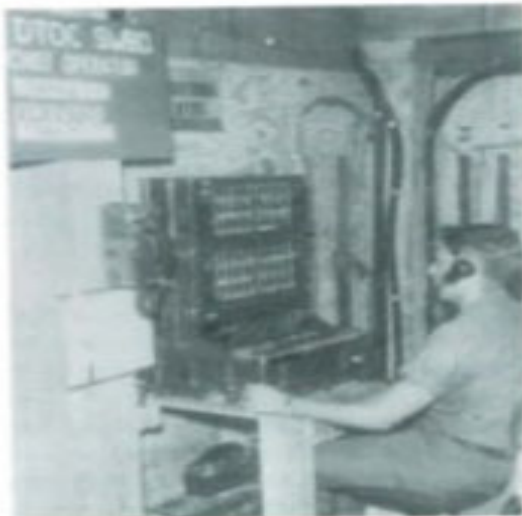
DIVISION TACTICAL OPERATIONS CENTER SWITCHBOARD, 125th Signal Battalion, 25th Infantry Division.
