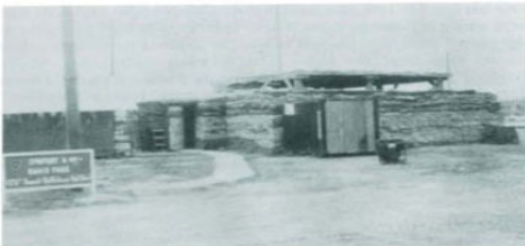
HIGH FREQUENCY RADIO BUNKER at 25th Infantry Division headquarters in Cu Chi. Antenna mast was made from artillery power canisters.
