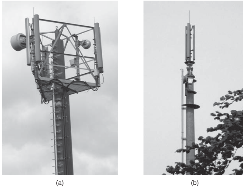
Figure 2.20 (a) Space diversity and (b) polarization diversity high-band antenna systems mounted on monopoles typically 15-m high (Photos by the author)
