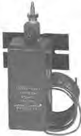
Figure 2.6 One-pipe capillary transmitter. (Courtesy of Johnson Controls Inc.)
