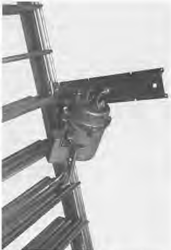
Figure 3.8 Frame mounted piston damper motor. (Courtesy of Johnson Controls Inc.)
