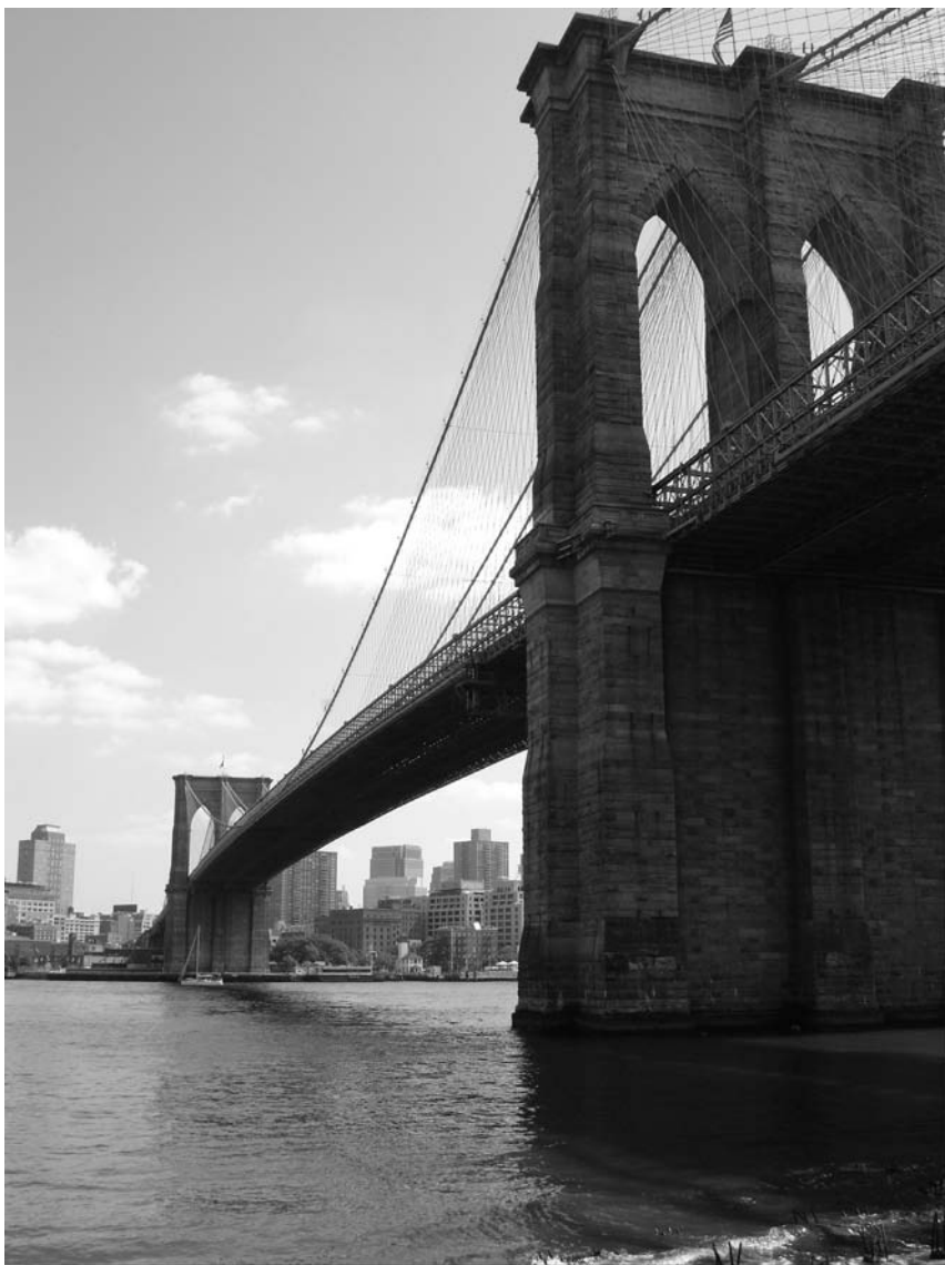
FIGURE 1-1: The Brooklyn Bridge from its base.
