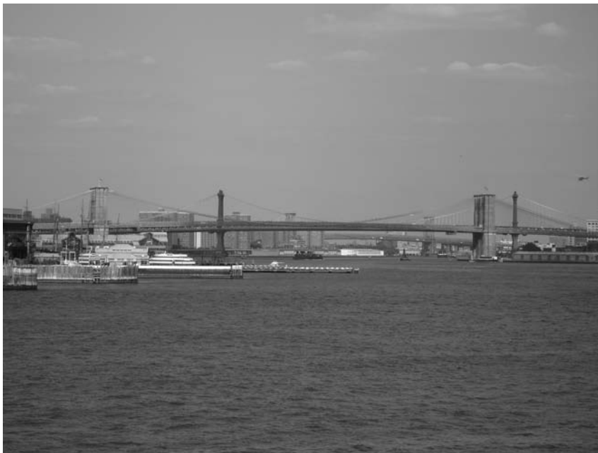
FIGURE 1-2: The Brooklyn Bridge from the Staten Island Ferry.
