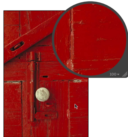
After Repair adjustment
