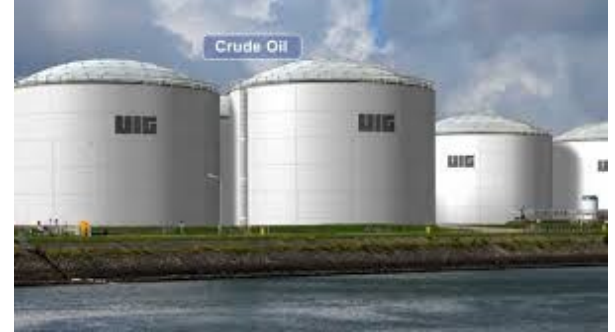
Clay’s field: oil storage
