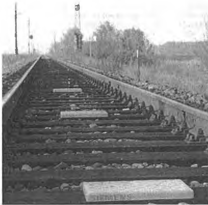
Figure 13.15: EURO-Balise in practical operation. (Reproduced by permission of Siemens Verkehrstechnik, Braunschweig)
