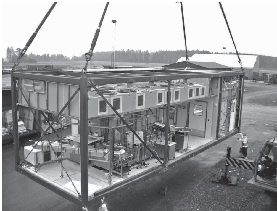
Figure 14-5 Example of a modular unit for a sterile manufacturing facility. Source: Courtesy of Pharmadule, Inc.
