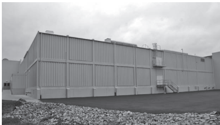
Figure 14-6 Exterior view of sterile manufacturing facility comprised of modular units. Source: Courtesy of Baxter Healthcare Corporation.
