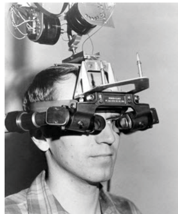
The Head-mounted Display (aka The Sword of Damocles) worn by Donald L. Vickers, one of Ivan E. Sutherland's Students at The University of Utah. Photo courtesy of Ivan Sutherland.
