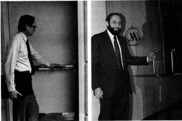
1.5 Affordances of Doors. Door hardware can signal whether to push or pull without signs. The flat horizontal bar A (above left) affords no operations except pushing: it is excellent hardware for a door that must be pushed to be opened. The door in B (above right) has a different kind of bar on each side, one relatively small and vertical to signify a pull, the other relatively large and horizontal to signify a push. Both bars support the affordance of grasping: size and position specify whether the grasp is used to push or pull—though ambiguously.
