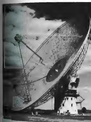
Figure 5.44 A paraboloidal radio antenna. (Photo courtesy of the Communications News and Information Bureau.)
