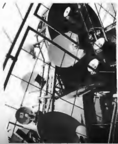
Microwave antennae on the top of the Eiffel Tower in Paris. (Photo by E.H.)
