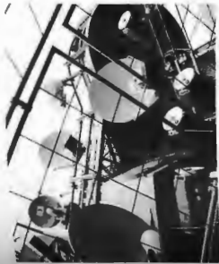
Microwave antennae on the top of the Eiffel Tower in Paris. (Photo by E.H.)
