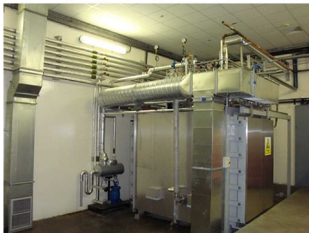
Fig. 3. Abbott Vascular two-pallet EO chamber
