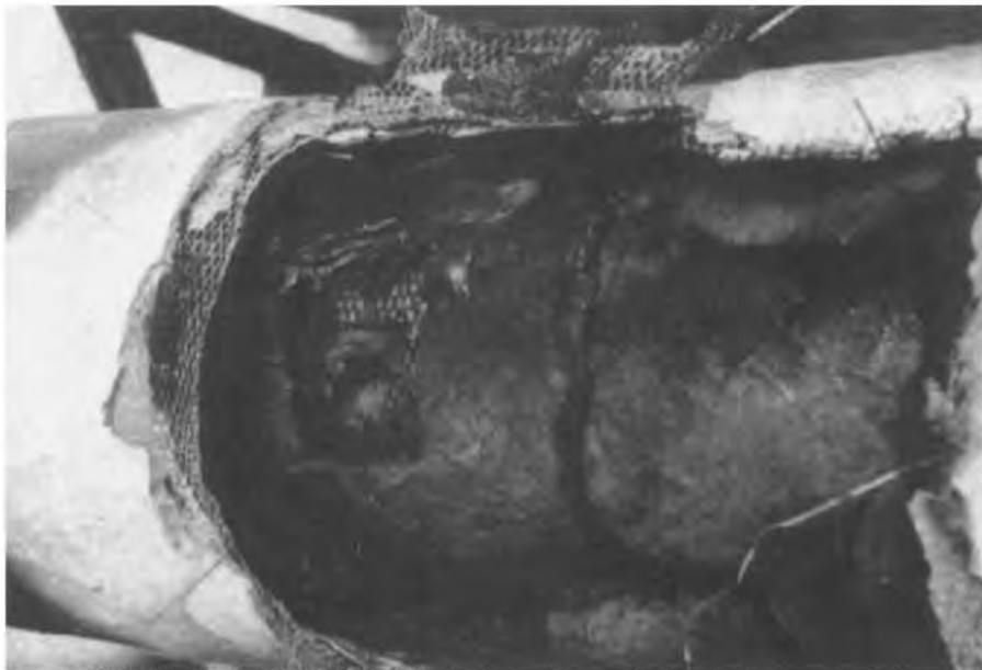
Figure 46. Results of fire test of a composite composed of U-modified isocyanurate foam and mortar (79). (Courtesy of Nisshin Spinning Co. Ltd.)
