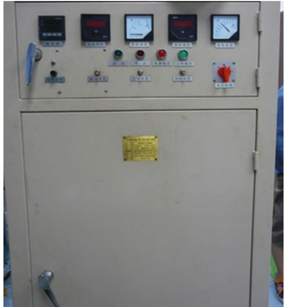
Fig. 6.1 AC electropulsing generator
