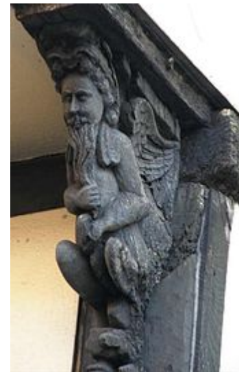
Brackets are used in traditional timber framing, including the support of a jettied floor which can be carved. Magdalene Street, Cambridge, England. Sixteenth century
