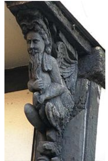
Brackets are used in traditional timber framing, including the support of a jettied floor which can be carved. Magdalene Street, Cambridge, England. Sixteenth century
