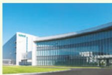
Pharmaceutical plant at the Kanto Factory
