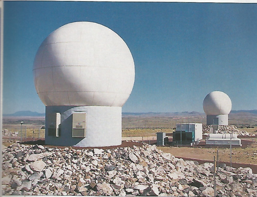
These 30-foot-tall Orbcomm gateway earth station antennas, located in the Arizona desert, provide communications links between the passing Orbcomm satellites and the network control center in Dulles, VA.
