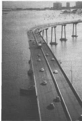
Figure 11-3. The Quickchange® Moveable Barrier system uses buried-wire guidepath control to automatically relocate concrete barrier sections on San Diego's Coronado Bridge for optimal lane usage during rush-hour traffic (courtesy Barrier Systems, Inc.).
