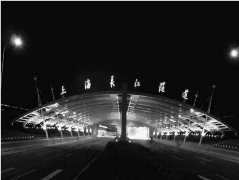
Figure 1.2 LED tunnel lighting in Shanghai Changjiang River Tunnel, China. (Reproduced with permission from www.gd-realfaith.com , Guangdong Real Faith Enterprises Group Co., Ltd., accessed April 12, 2011.)
