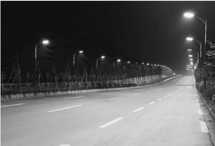
Figure 1.4 LED road lighting in Guangdong Province, China. (Reproduced with permission from www.gd-realfaith.com , Guangdong Real Faith Enterprises Group Co., Ltd., accessed April 12, 2011.)
