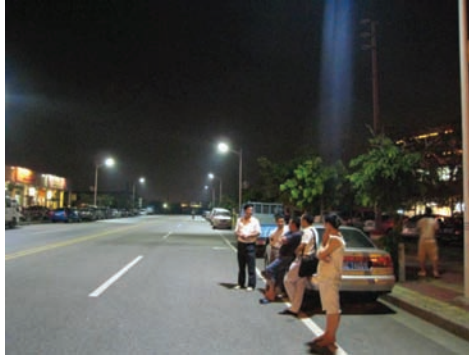
Figure 6.55 Actual illumination performance of the 112W LED road lights at Meishi Street, Nanhai District, Foshan City, Guangdong Province, China. (Reproduced with permission from www.gd-realfait.com , Guangdong Real Faith Enterprises Group Co., Ltd., accessed April 12, 2011.) ( Color version of this figure is available online. )
