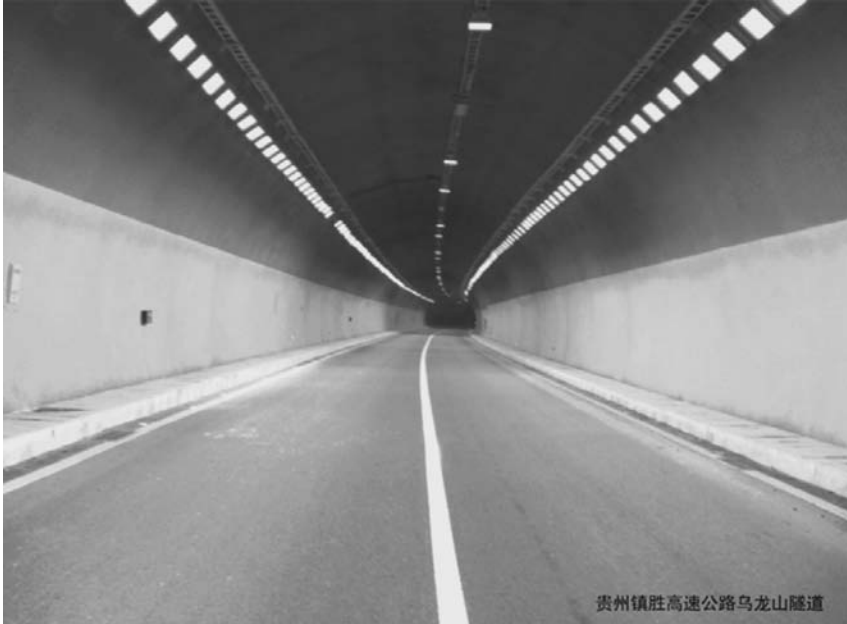
Figure 1.3 LED tunnel lighting in Guizhou Province, China. (Reproduced with permission from www.gd-realfaith.com , Guangdong Real Faith Enterprises Group Co., Ltd., accessed April 12, 2011.)
