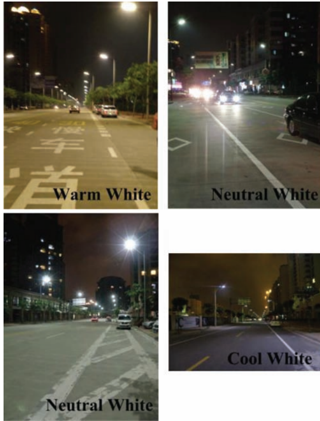
Figure 6.99 Road illumination performance of LED lamps with different color temperatures at Meishi Street, Nanhai District, Foshan City, Guangdong Province, China. ( Color version of this figure is available online. )
