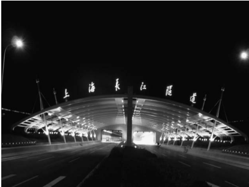
Figure 1.2 LED tunnel lighting in Shanghai Changjiang River Tunnel, China. (Reproduced with permission from www.gd-realfait.com , Guangdong Real Faith Enterprises Group Co., Ltd., accessed April 12, 2011.)
