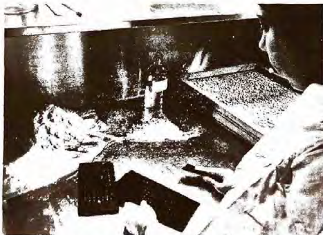
Fig 33. Hand-molding tablet triturates (courtesy, MSD).
