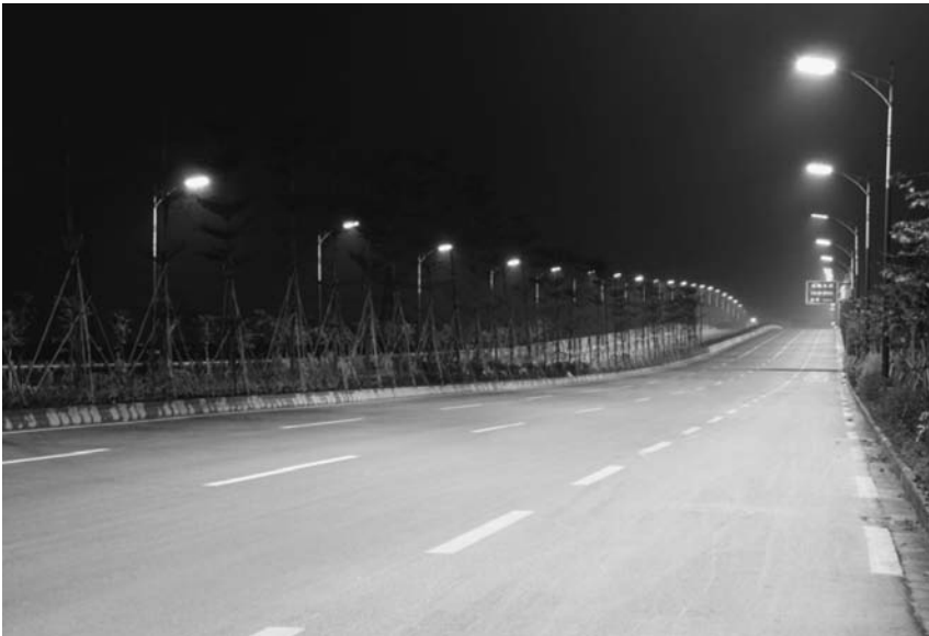
Figure 1.4 LED road lighting in Guangdong Province, China. (Reproduced with permission from www.gd-realfait.com , Guangdong Real Faith Enterprises Group Co., Ltd., accessed April 12, 2011.)
