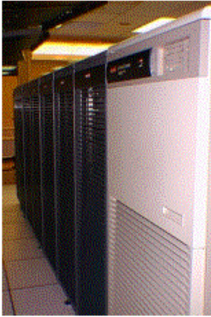
Figure 1. The TerraServer hardware
