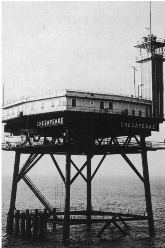
Figure 501a. Typical offshore light station.
