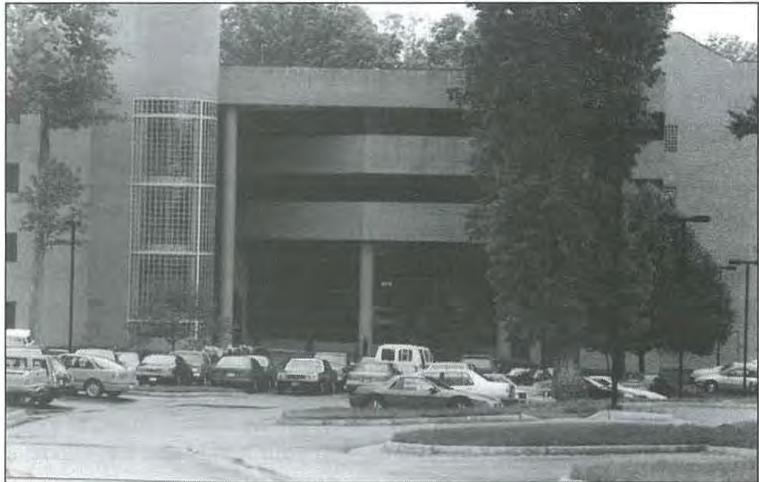
Figure 1-1: America Online nestles snugly in this office building in the Virginia forests just outside Washington, DC.
