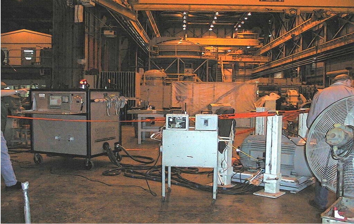
PHOTO SHOWING THE ADM AND RADIO MODEM IN USE AT TVA'S POWER SERVICE SHOPS
