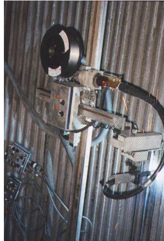
Automated Waterwall Tooling (4-6 times manual production)
