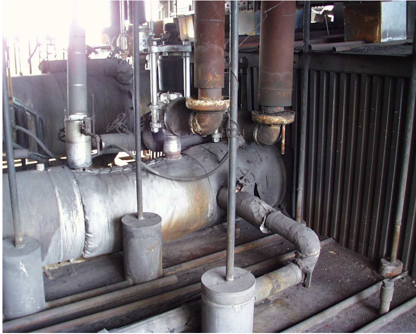
Figure 5. Plant A Main Steam Outlet Terminal Header Inspection Location
