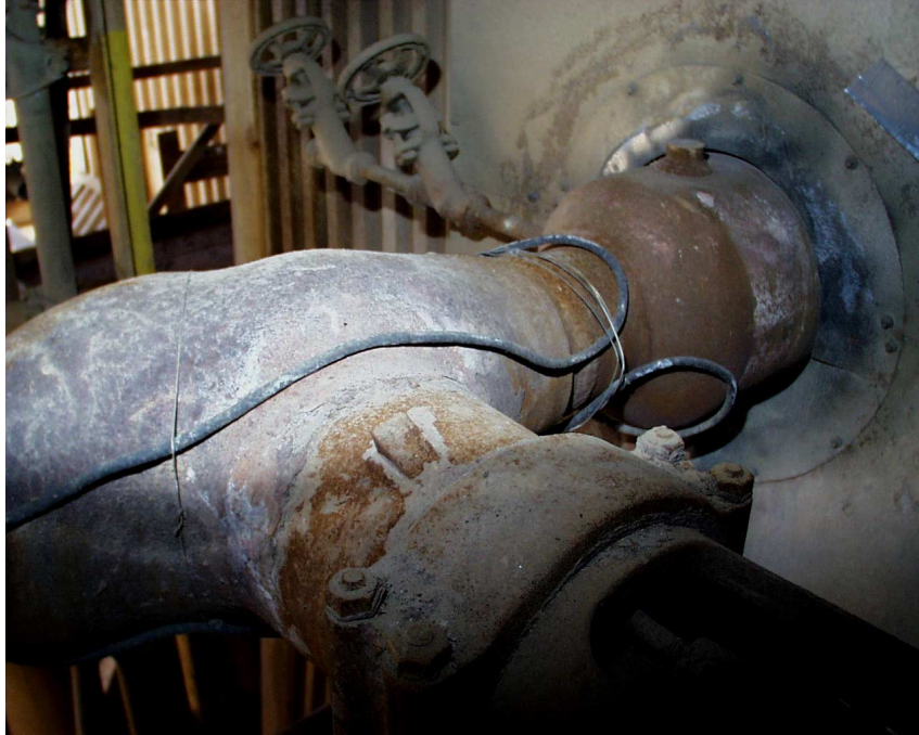
Figure 7. Plant B Feedwater Piping – Economizer Inlet – Prepped for UT Inspection
