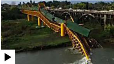
▶ Chile bridge collapses as train crosses
