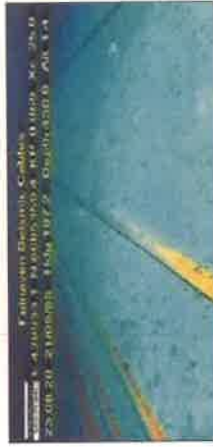
Fig. A2. Hydrophone cables laid in position on the seabed over Foinaven Field, west of Shetland. To make sure that strong currents did not move the cables (which would have affected the repeatability of the survey), they were buried in a seabed trench that was dug using a water jet from a remotely operated vehicle—technology routinely applied to transoceanic power and telecommunications cables.
