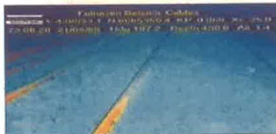
Fig. A2. Hydrophone cables laid in position on the seabed over Folnaveen Field, west of Shetland. To make sure that strong currents did not move the cables (which would have affected the repeatability of the survey), they were buried in a seabed trench that was dug using a water jet from a remotely operated vehicle—technology routinely applied to transoceanic power and telecommunications cables.
