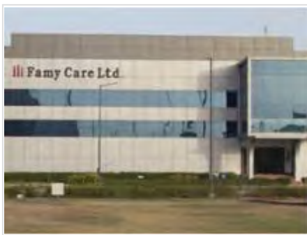
Famy Care's Ahmedabad plant
