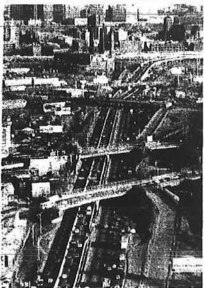
TRAFFIC IS MOVING — Cars move along South Street Expressway during rush hour traffic Monday, the first day of reconstruction on the busy highway connecting southeastern Massachusetts and communities with Boston. Expected major delays failed to occur. (AP Photo)
