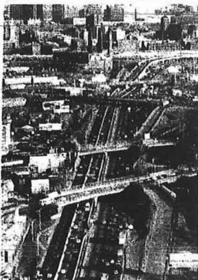
TRAFFIC IS MOVING — Cars move along South Street Expressway during rush hour traffic Monday, the first day of reconstruction on the busy highway connecting southeastern Massachusetts and communities with Boston. Expected major delays failed to occur. (AP Photo)
