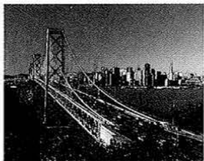
suspension bridge San Francisco-Oakland Bay Bridge
