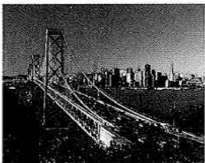
suspension bridge San Francisco-Oakland Bay Bridge
