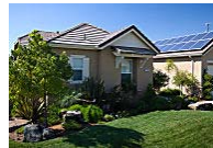
Thinking about getting Solar Panels? Read This First Solar America
