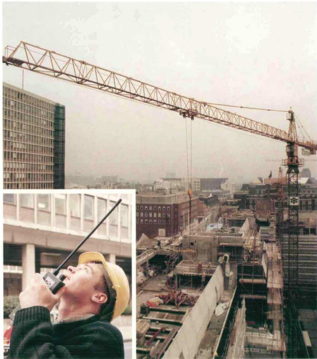
Portable radio for safety work between the ground and a tower crane
