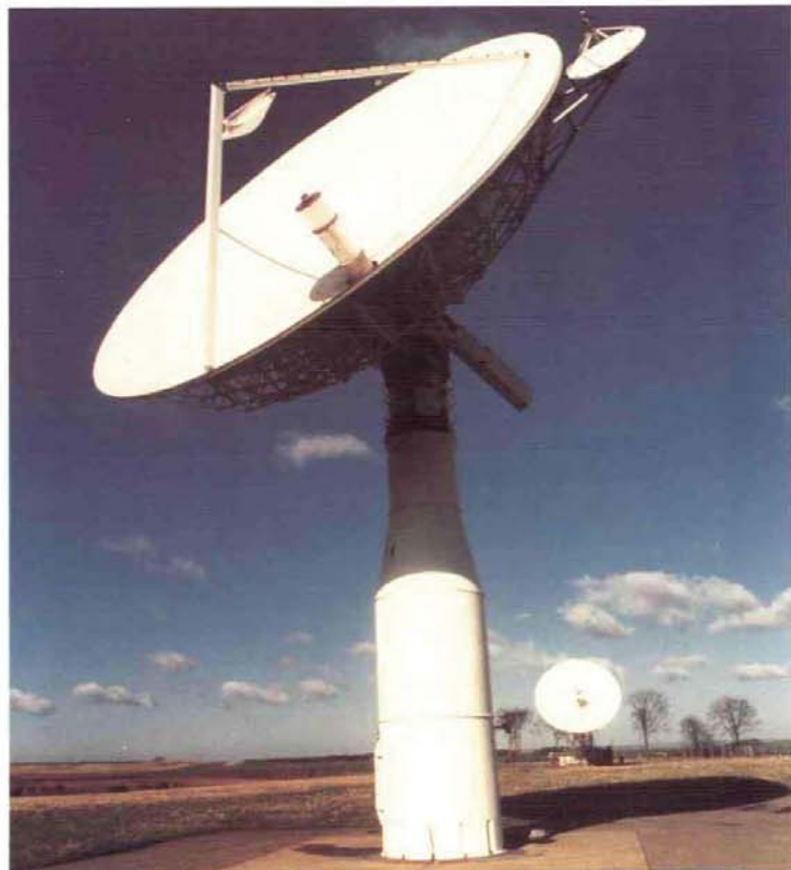
The Satellite Monitoring Station at Ballock
